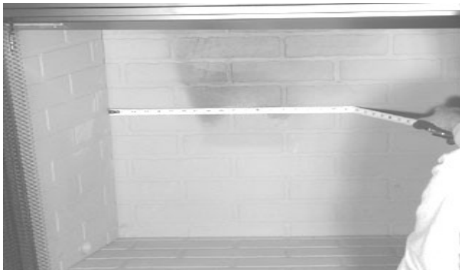
Figure 1 Measure Firebox
