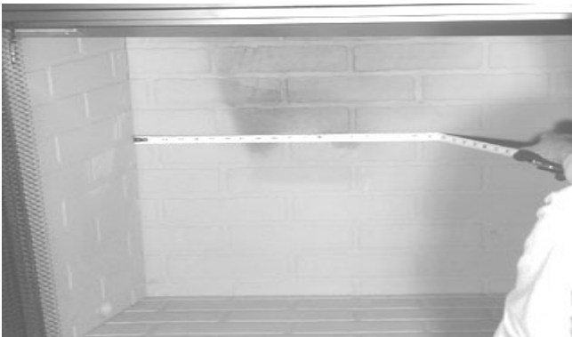
Figure 1 Measure Firebox
