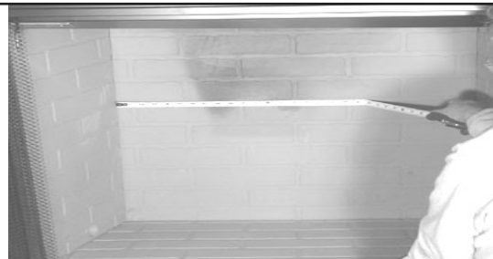
Figure 1 Measure Firebox
