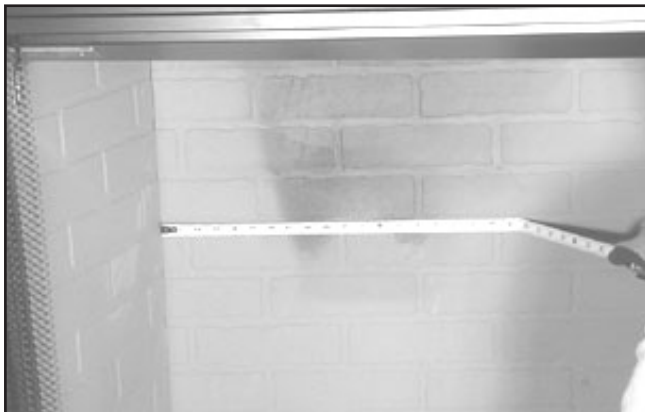
Figure 2.1 Measure Firebox
